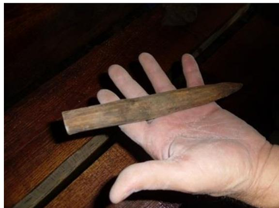
The original post and beam construction was revealed, and the pegs used in construction were found.
