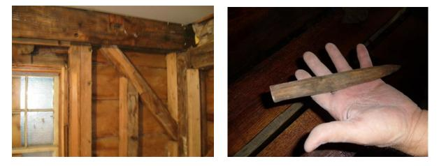
The original post and beam construction was revealed, and the pegs used in construction were found.
